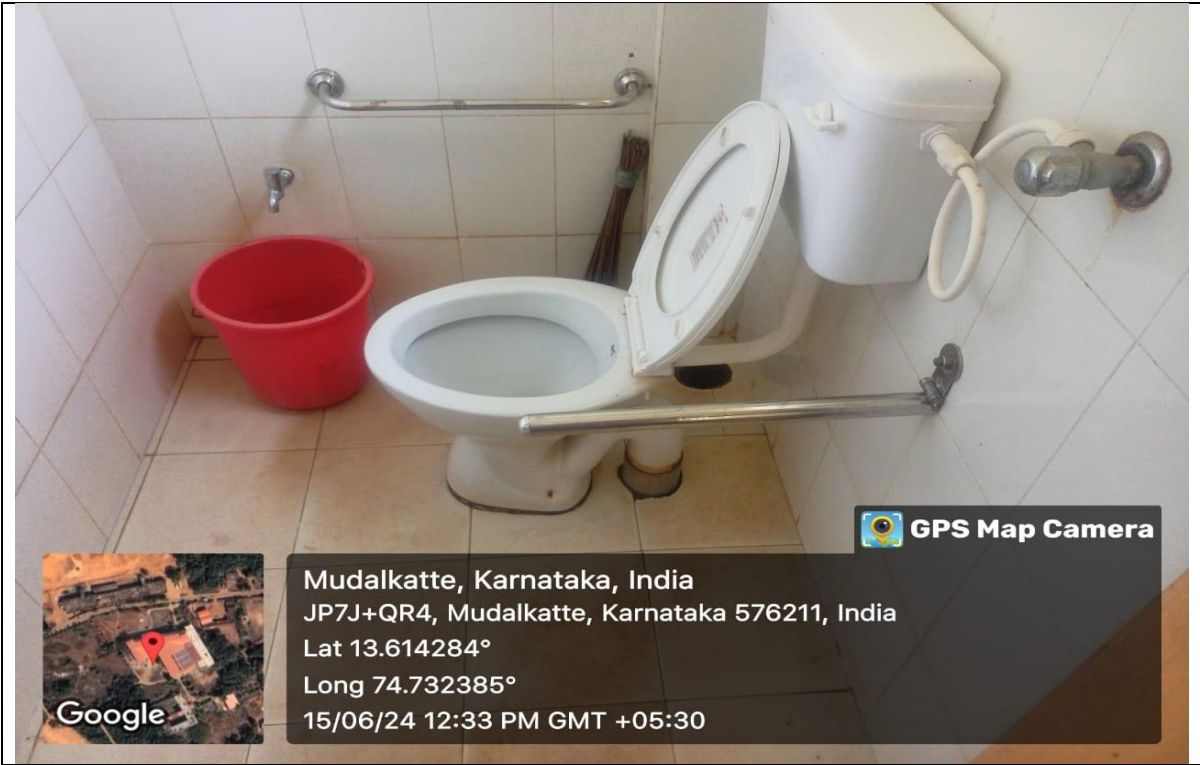
Washroom for disabled
